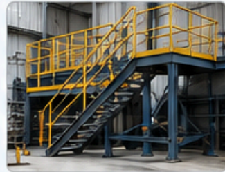
Platforms, Ladders, Handrails & Walkways
