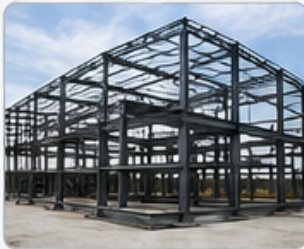
Structural Steel Fabrication
